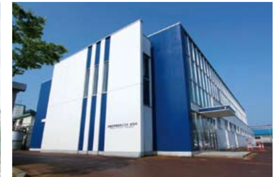
H Central Research Laboratory (Nagaoka City, Niigata Prefecture)
