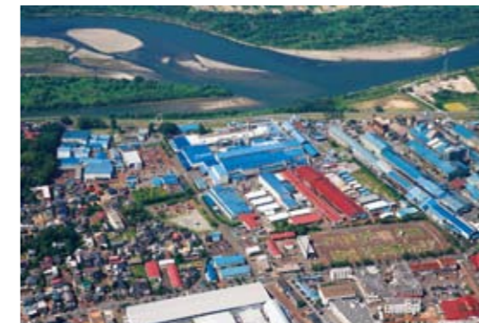
E Nagaoka Mill (Nagaoka City, Niigata Prefecture)
