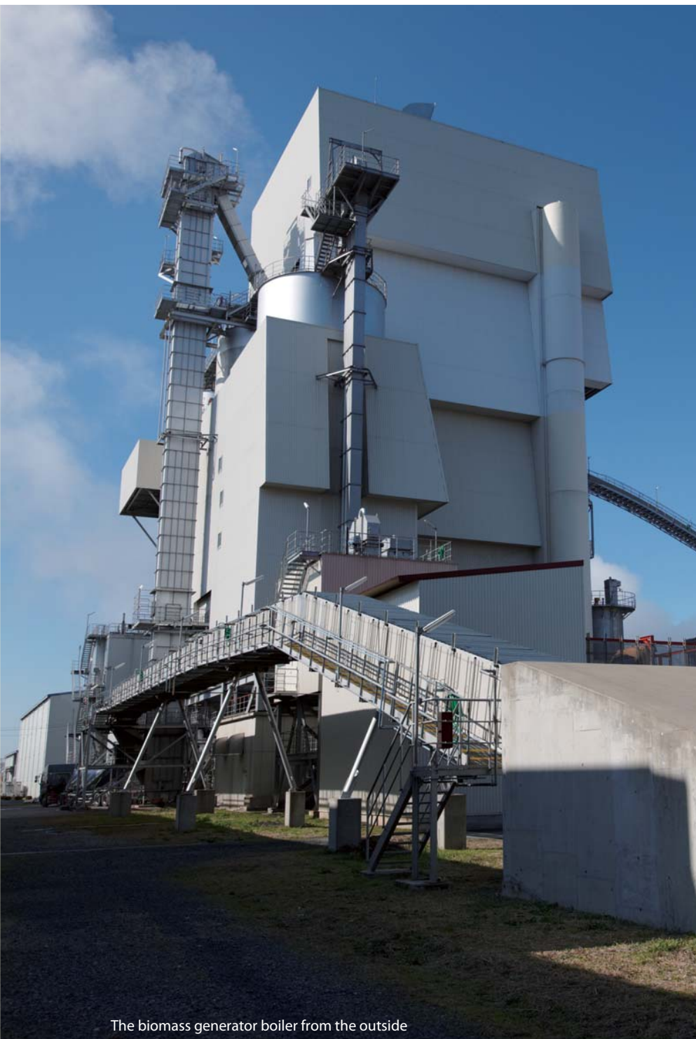
Wood-fuel pulverized for fuel being carried to the boiler
