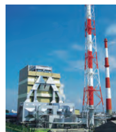
Niigata Mill Black liquor recovery boiler
