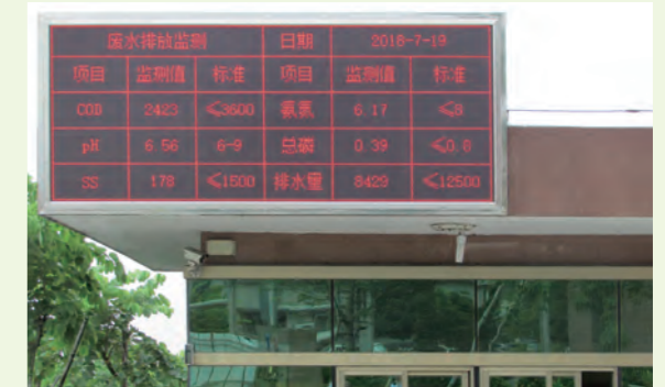
Electronic bulletin board installed at the front entrance with a live display of environmental values
