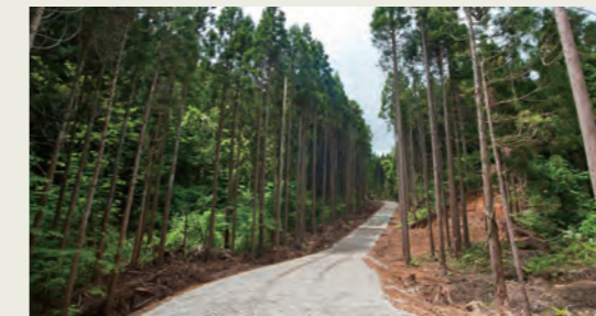
A forestry road in a company-owned forest in the Anamizu area constructed by local companies using grant money.
