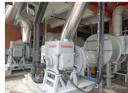
Jiangmen Xinghui Paper Manufacturing Linear Vacuum Pump (Achieves 37% energy savings compared to existing equipment)
