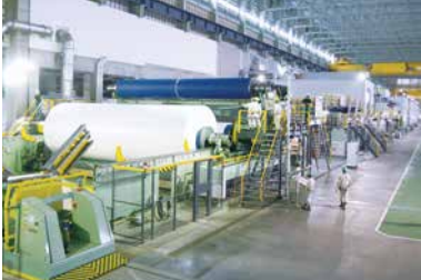
The No. 9 paper machine at the Niigata Mill, a massive 223 meters in length, carries out integrated processes from base paper making to coating to produce roll paper with a width of 10m and a length of 180km.
