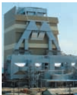
2004年新設の8号回収ボイラー The No. 8 recovery boiler, newly constructed in 2004
